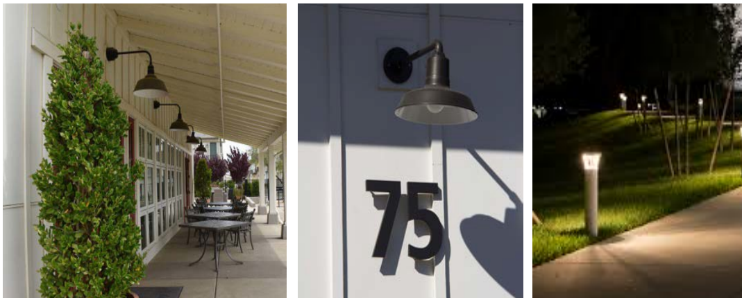
Gooseneck Light fixtures illuminates a porch; Addresses should be illuminated for easy wayfinding and safety; pathway lighting should direct visitors to entries and provide safety.
