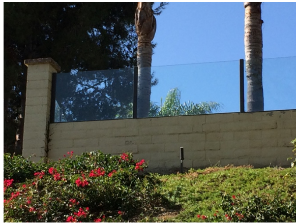
Masonry and Glass View Wall
