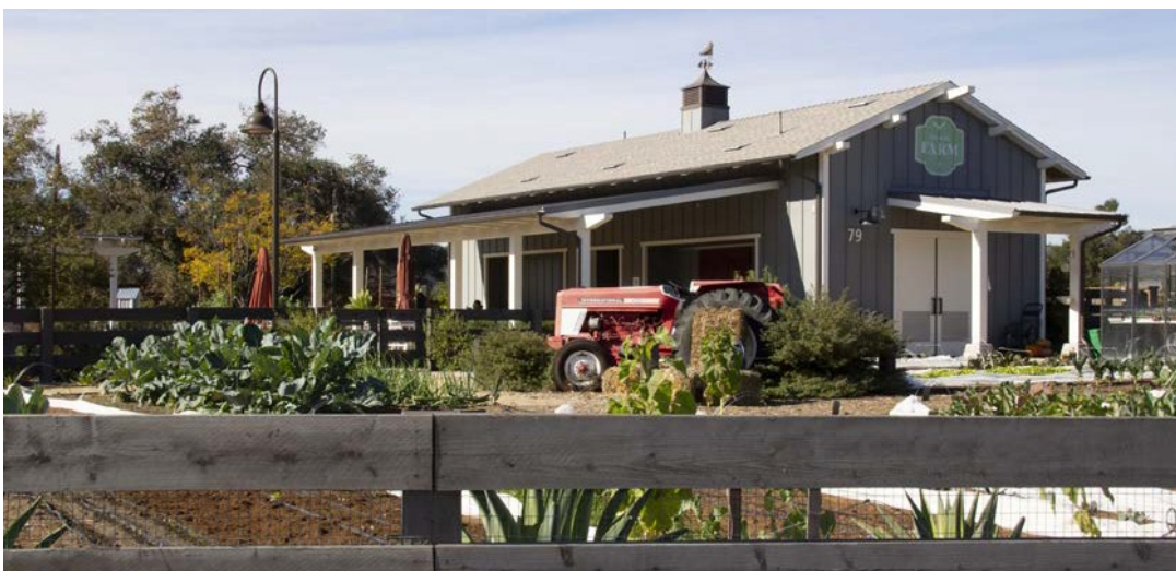
Buildings should be designed to resemble those that would be found on a farm or ranch.
