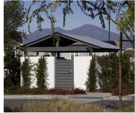
Covered trash enclosures protect refuse from stormwater and prevent pollution from entering the storm drain system.
