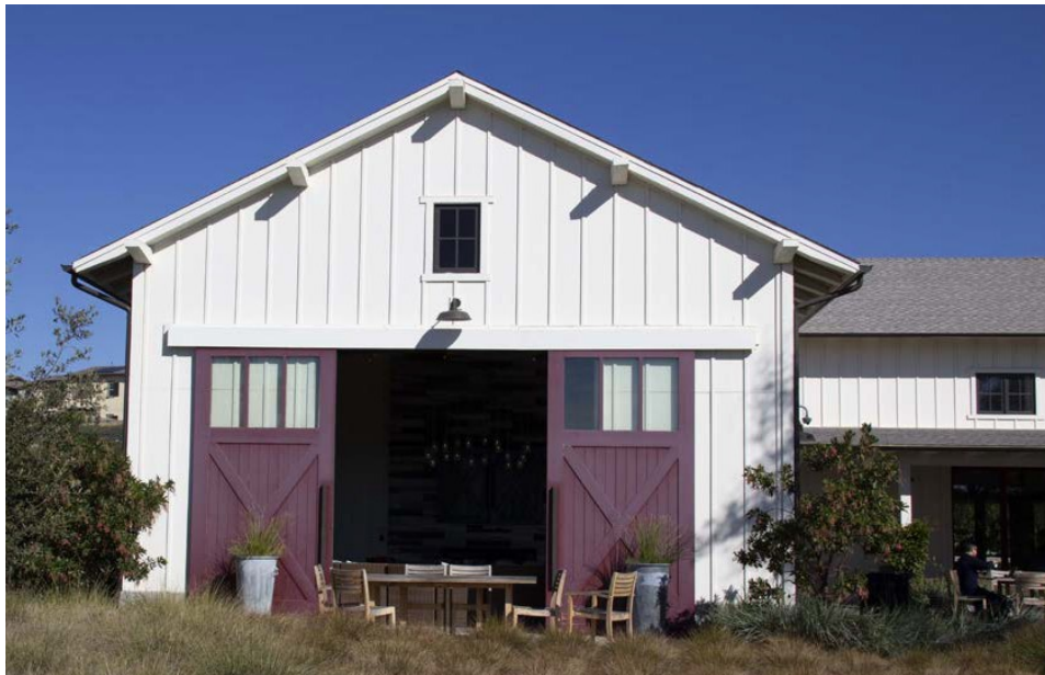
Sliding barn doors are a common feature in farm buildings and provide excellent indoor-outdoor connectivity.
